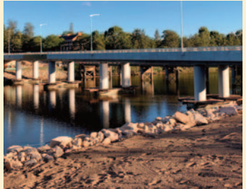
The New Windsor Bridge – on track for completion
